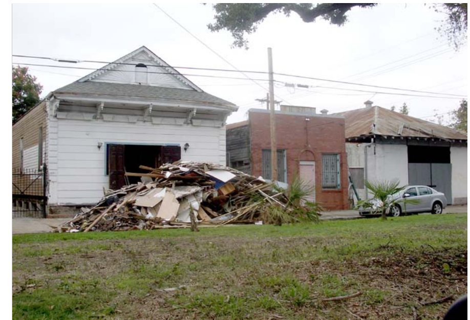
Demolition debris in Bywater.
